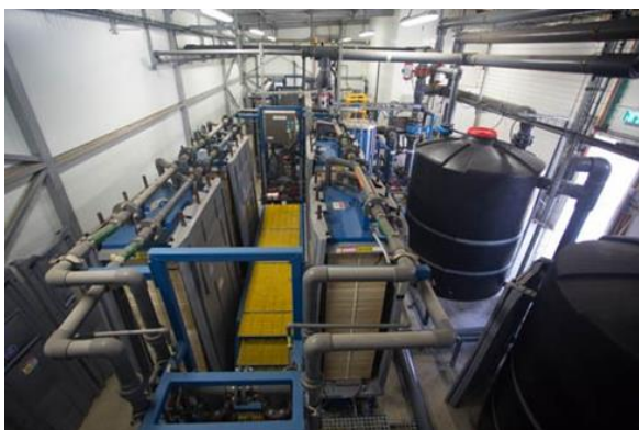
Figure 1: Veolia's EDR system installed at Kfar Saba
