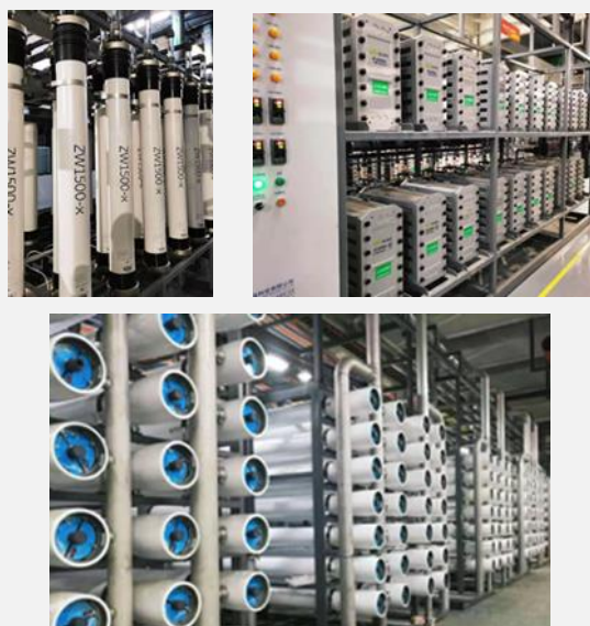
Figure 2: Membranes used in this project -- ZeeWeed UF (left), E-Cell EDI (right) and RO System (bottom)
